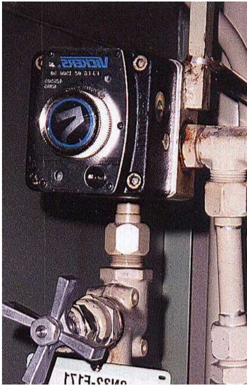
Showing Vickers Flow Control Valve. Key slot is to lower right.
