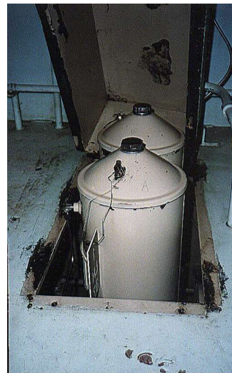
Showing long housings extending up thru the deck. Takes 4 '718' cartridges.
